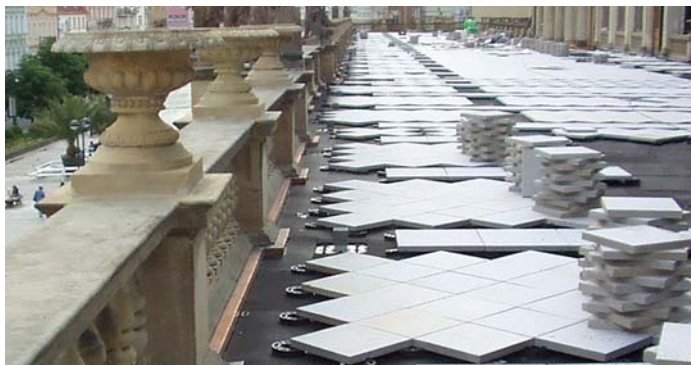
Mill Colonnade , Karlovy Vary – design documents and author's supervision in the restoration of the high-reliability composite insulation of a terrace (double waterproofing system).
